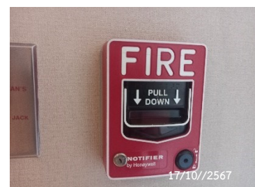
Fire Alarm Manual Station
